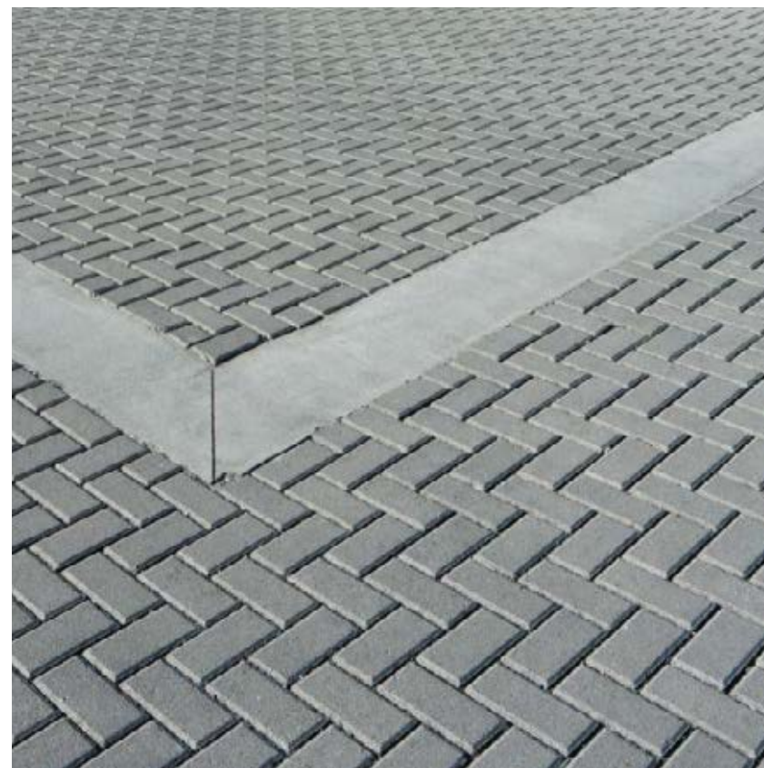
5. THRESHOLD PAVING / Holland firth pavers, Herringbone patterns, header coarse
