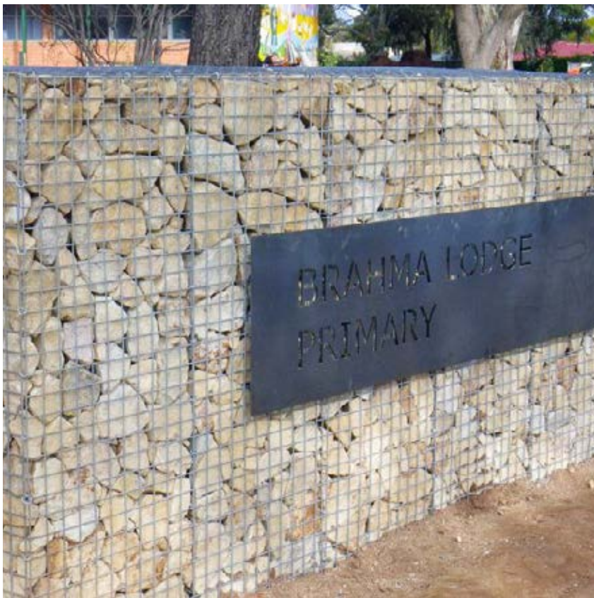
3. MATERIALS TO ENTRY AREA / Gabion stone walls, Corten steel panels, Signage, Timber posts /
