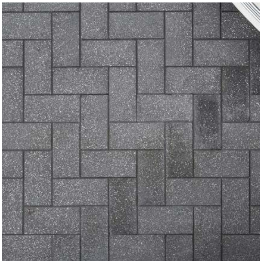
5. THRESHOLD PAVING / Holland firth pavers, Herringbone patterns, header coarse
